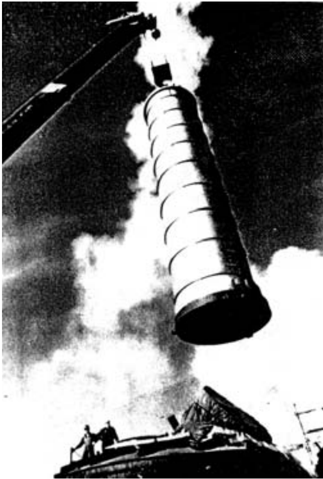
A type 316L "candle" for a radial flow converter. The candle was loaded in a weatherproof loading area to keep both it and the catalyst free from moisture. Shown fully charged here, it is being lifted to the top of the converter for installation through the manway.
