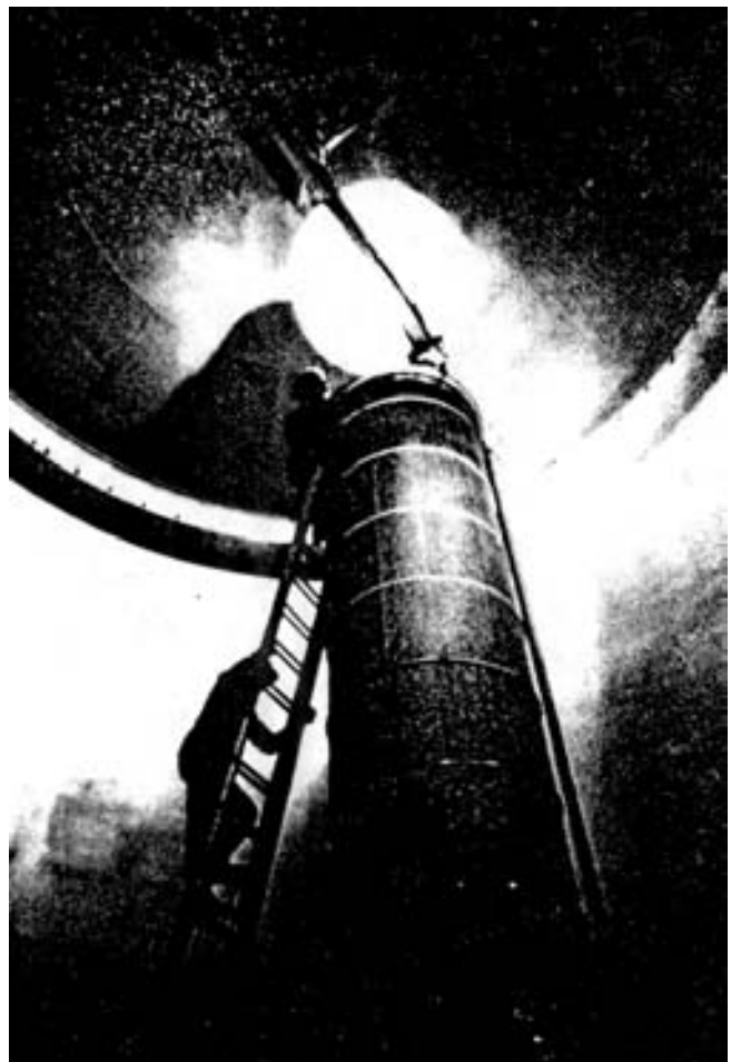
The first of several Type 316L stainless steel catalyst "candles" are placed in position within a radial flow converter.
