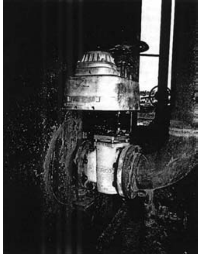
This DURIMET alloy 20 valve handles 93 percent H 2 SO 4 at ambient temperature.
